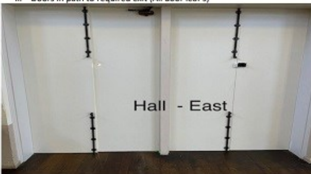
ii. Doors in path to required exit (All door leaf’s)
